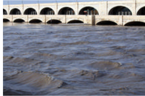
Flooding of Sukkur Barrage
