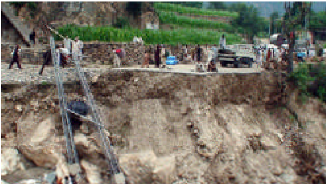
Landsliding on Karakoram Highway
